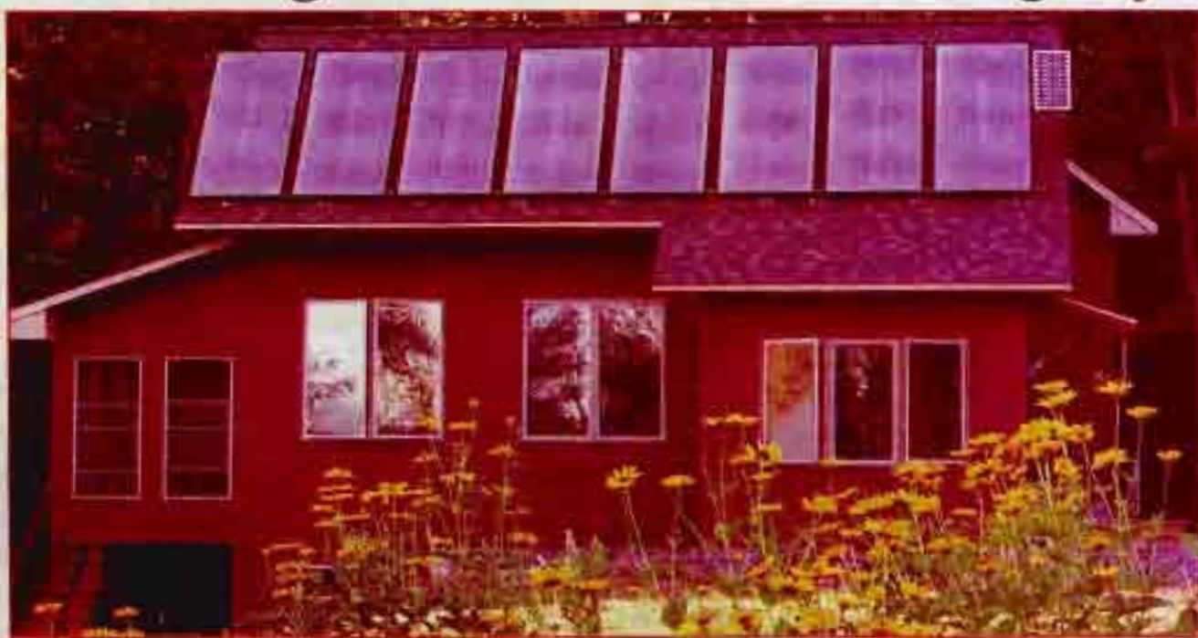
The solar panels on top of this cabin provide the occupants with year-round heating and hot water while blending in with the surrounding foliage.. Special Photo.
